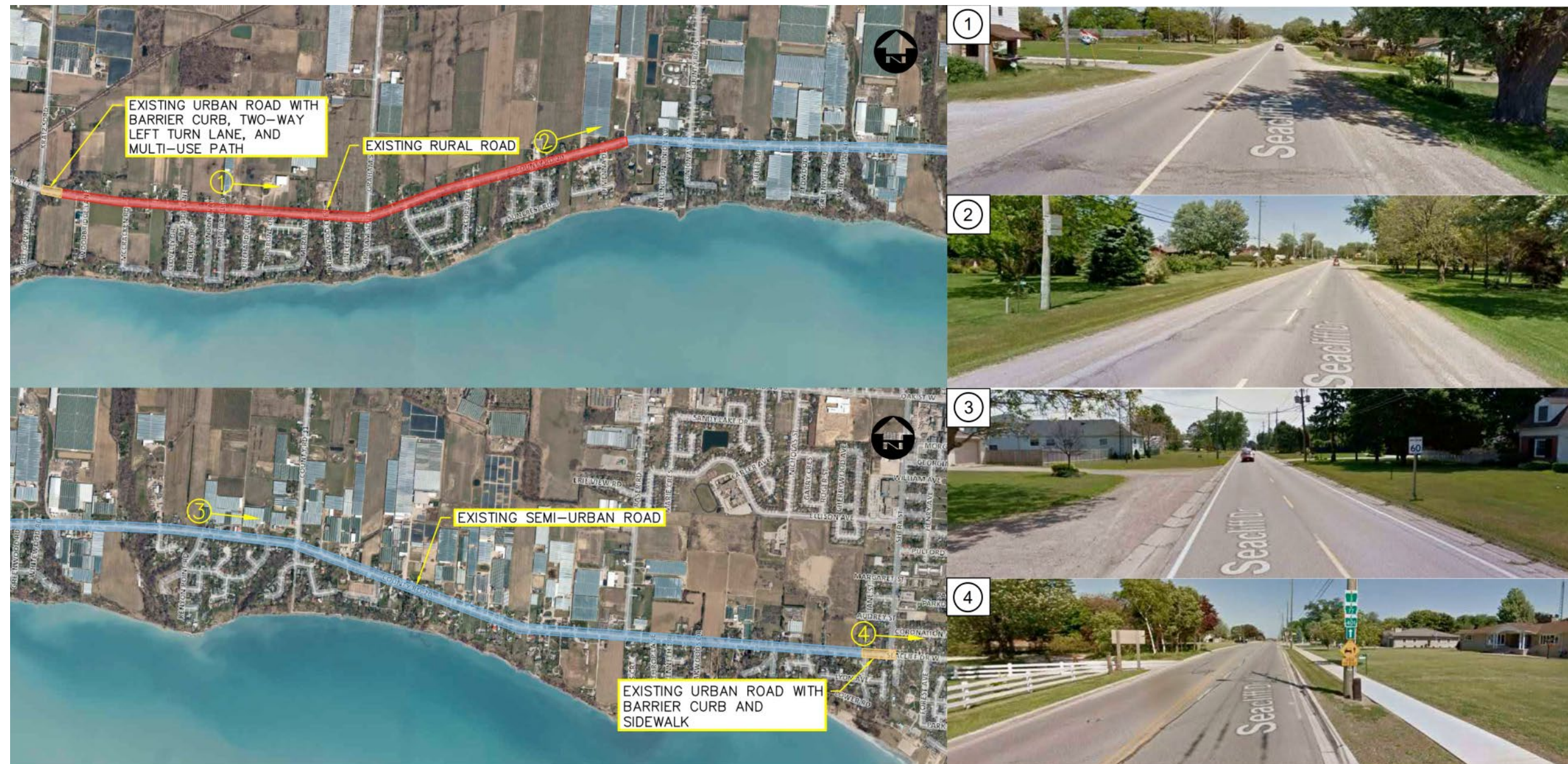
Figure 7: Existing Road Conditions
